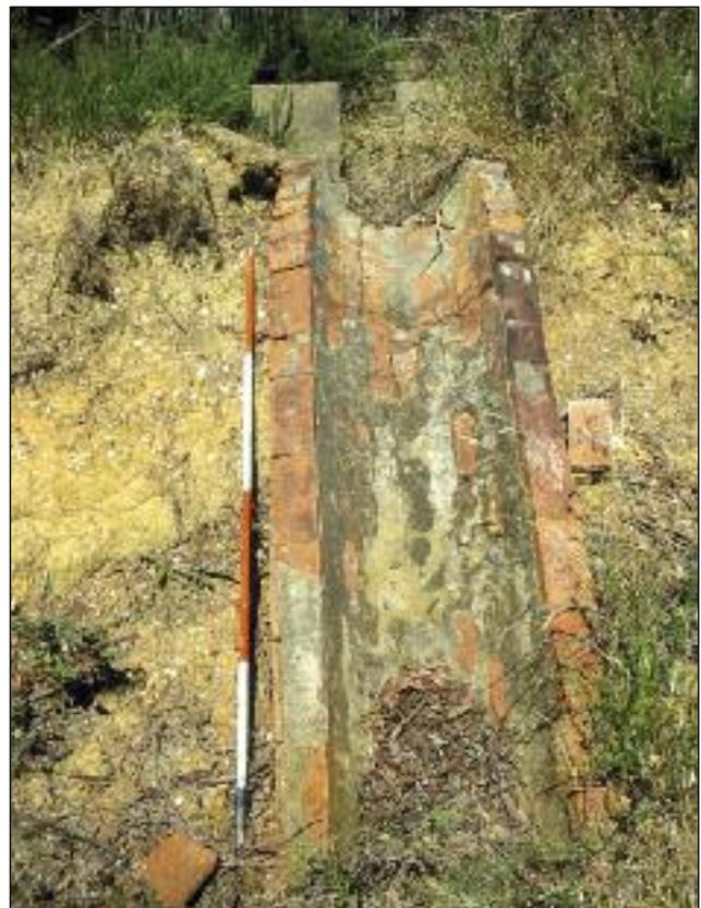
Figure 6: Brick-lined sluice from Humbug race into Lincoln Gully Reservoir (Davies 2012).
