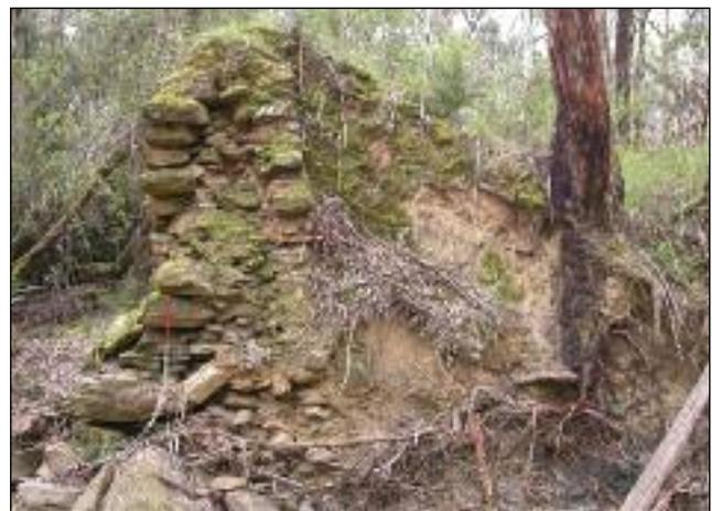
Figure 3: North section of Eatons Dam, breached by flooding in 1933 (Davies 2011).
