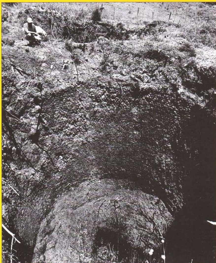
Kiln 1 at Victoria battery in January 1997, showing brick lining and entrance to the ore chute, at bottom.
