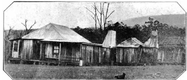
Figure 4: Billy Maxwell's huts on portion 1, Kedumba parish, photographed in 1927 from the east. The southern end of his 1893 hut, still with a bark roof, is on the far right, behind the cooking shed of 1894, reclad with a corrugated metal roof. The 1925 hut, which survives, with its skillion extension and chimney of 1926 on the north, occupies the left half of the image (*Daily Guardian*, 10 January 1927:7).
