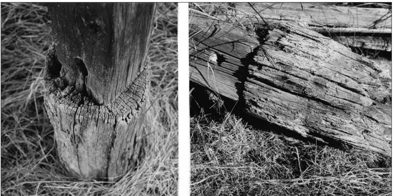
Figure 8: Two very similar corner posts, both hewn square by Billy Maxwell from round timber embedded in the ground. The post on the left belongs to the 1925 hut, the post on the right to the ruins of the 1893 hut nearby (Ian Jack, 2001).
