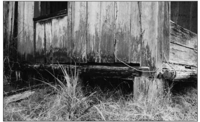
Figure 7: South-east corner of Billy Maxwell's 1925 hut, from south-east. The squared-off corner post is similar to the 1893 post shown in Figure 8. The south window uses part of the slab wall as its framework, while the horizontal sill, which has helped to preserve the hut, is held in place by mortise and tenon joints (Ian Jack, 2001).
