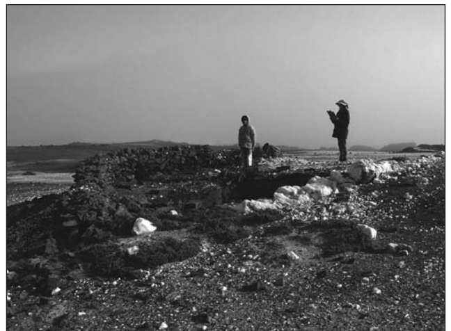
Figure 4: One of the Site 4 mine shafts, showing the quartz vein and curving drystone wall constructed from waste rock.
