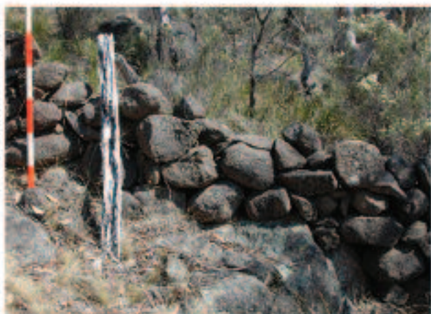
A truncated pair of dog-legs across a low part of the wall.
