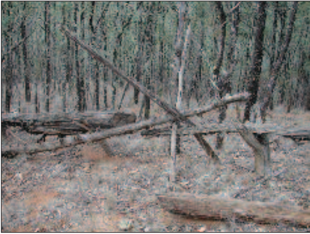
Figure 4a: Lateral view of dog-leg fence at Mt Trooper, south of Ingebyra, New South Wales, showing forked posts supporting logs laid head to butt. The second tier of logs rests in the crutch of the dog-legs, and one partly dislodged log remains. The log in the right foreground had been a second-tier log, but fell as the next pair of crossed poles collapsed.
