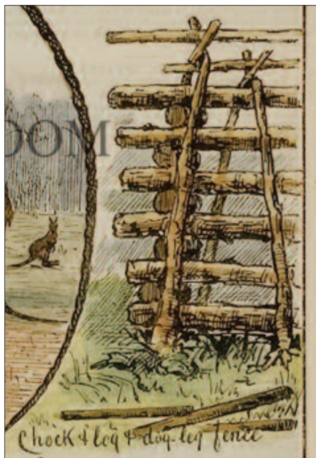
Figure 2: 'Chock & log & dog-leg fence' showing two sets of dog-legs or crossed poles increasing the height of the extremely high (and perhaps fanciful) chock-and-log fence, and supporting top rails or poles (The Antique Print Room).
