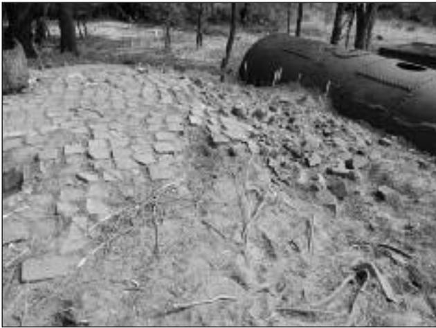
Figure 5: Cornish boiler and brick floor feature, with in situ post (top left). Several sections of the floor have collapsed due to heavy erosion.
