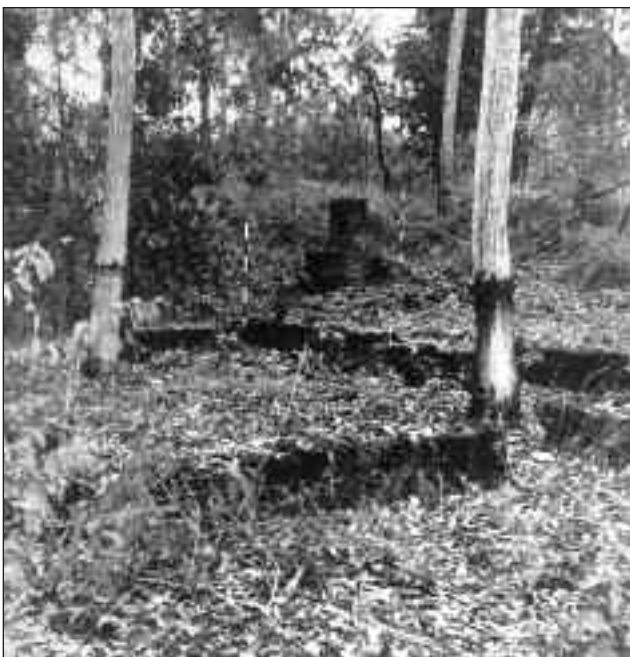
Figure 8. Foundations of the hospital (VH) in foreground, looking north-west towards the remains of the dispensary (VHD).
