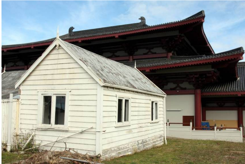
Stancombe Road Cottage (the Baverstock School additions) prior to removal and excavation, with the Buddhist Temple in the background
