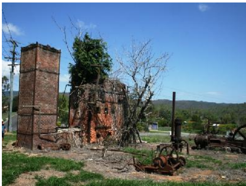
Remnants of the chimney, boiler and Marshall steam engine at Mount Molloy (Source: DERM)
