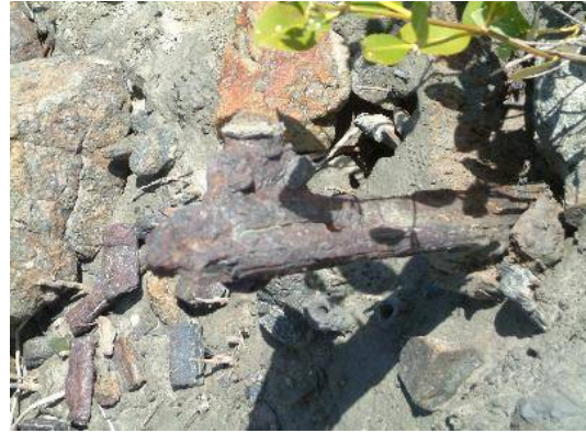
Corroded rail fragment, Habana causeway
