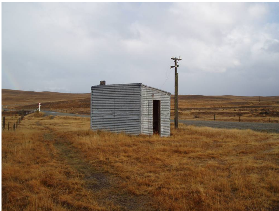
Plate 1: Braemar Road roadman's hut.
